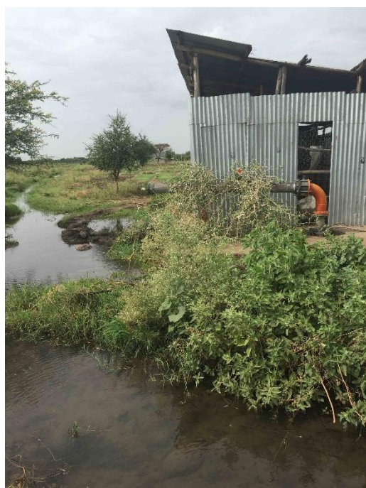
Figure 7. Borehole and canal for irrigating lands
